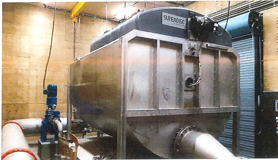
FIGURE 3-6: WESTECH SUPERDISC FILTER – CHASE WWTP
