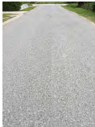
FIGURE 2-3: PAVEMENT EXAMPLES SHOWING FAIR CONDITION (5 - 7)
